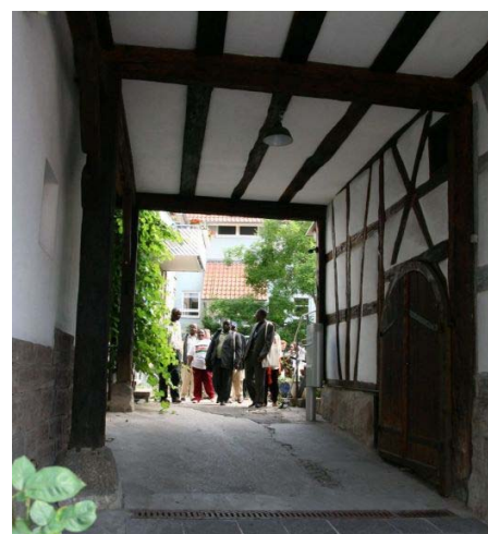
Archway at Rebmann House
